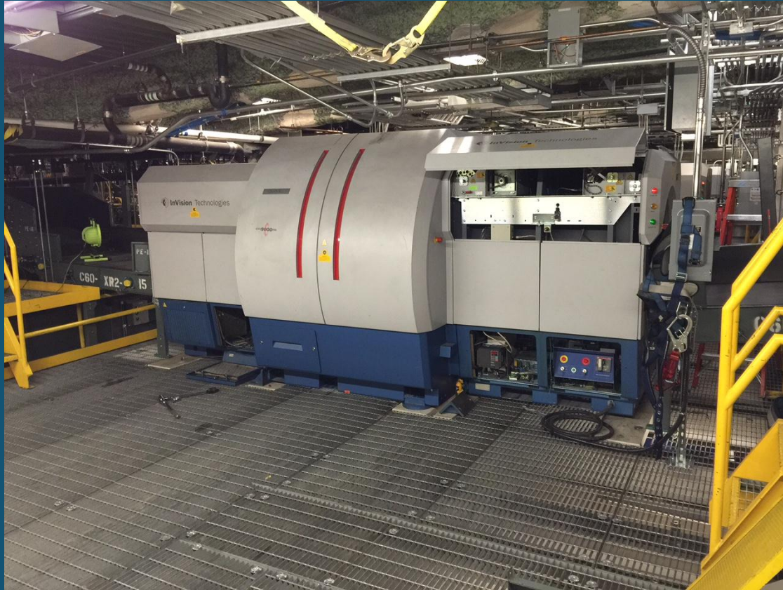
C60 and C61 BHS Modifications
