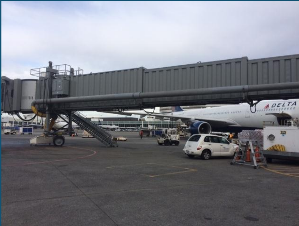
Passenger Loading Bridge – B14
