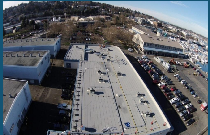
FT Nordby Roof
