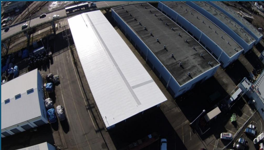
Net Shed 9 Roof
