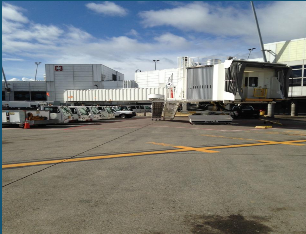
Passenger Loading Bridge – C3
